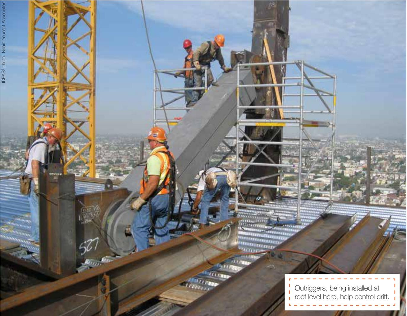
Outriggers, being installed at roof level here, help control drift.
